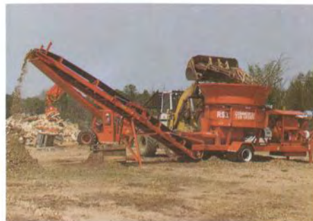
Pallets, slab wood and demolition debris
